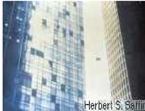
Windows falling from a high building.
