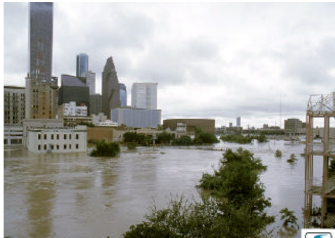
Inland flooding from Tropical Storm Allison in 2001
