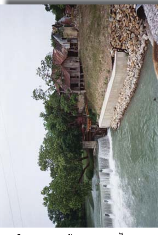
The City of Luling receives most of its water from the San Marcos River, shown here at the old Zedler Mill and Dam in Luling.
