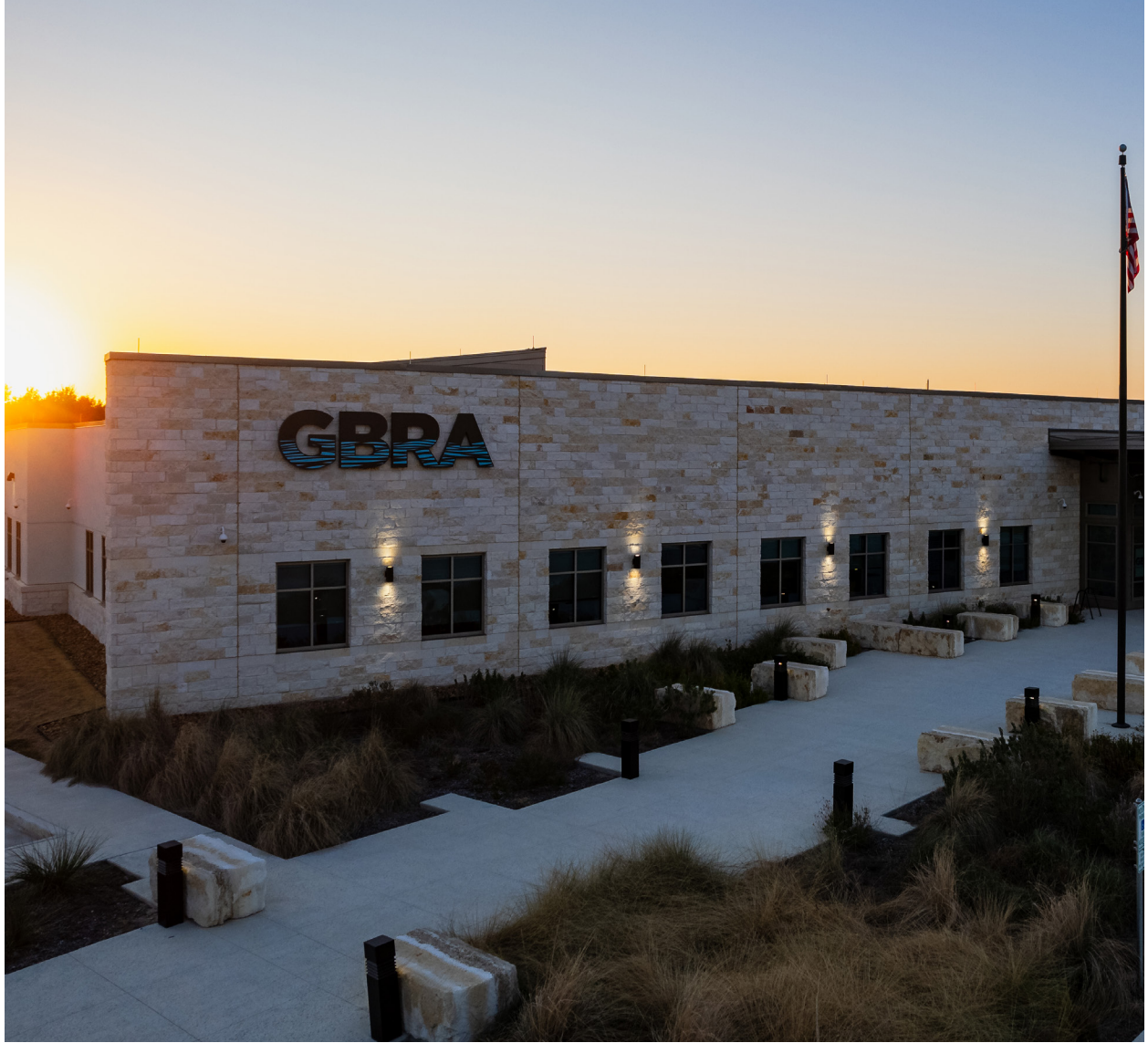
GBRA Headquarters in New Braunfels.
